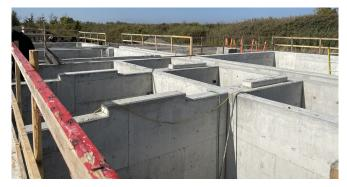
Xypex Admix C-500 provides integral waterproofing by forming a crystalline structure within the concrete, protecting it from the inside out and eliminating the need for external membranes or coatings.
